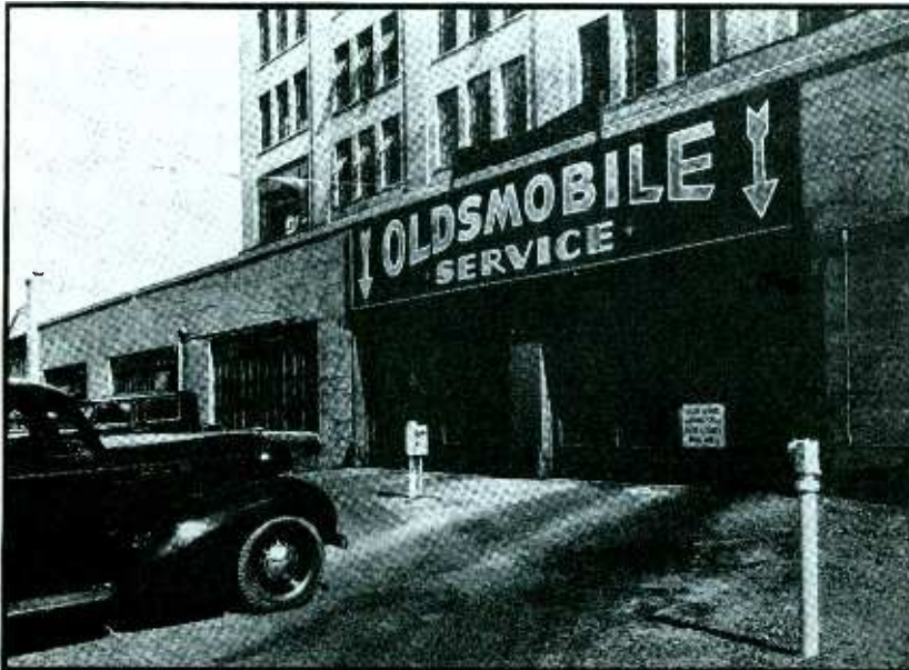
Fig. 3—Service garage entrance. Controls housed in water-tight case
